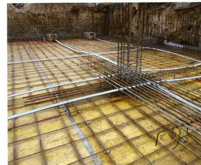
FIGURE 8.6-1 Grouted Slab (Morocco; P720)
