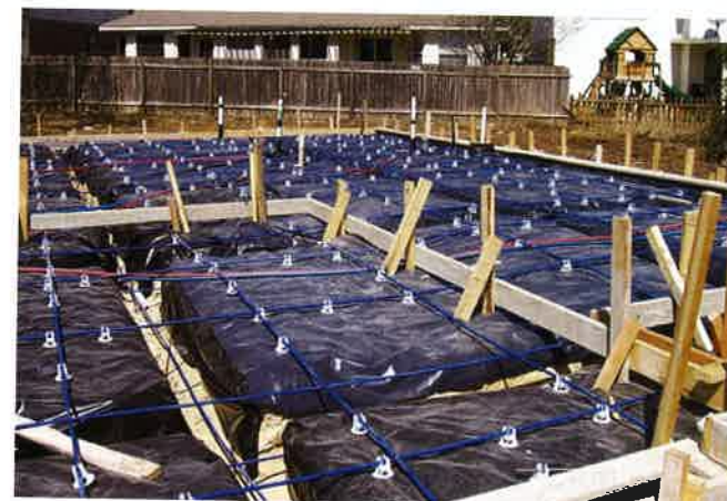
FIGURE 8.6-10 Unbonded Residential Foundation (US; P729)
