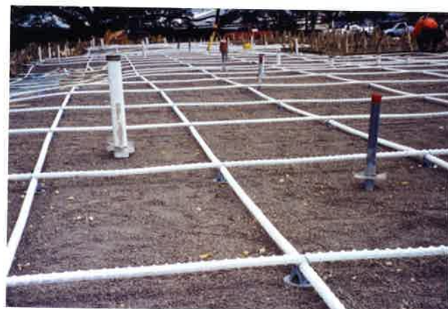
FIGURE 8.6-9 Grouted Residential Foundation (US; P728)
