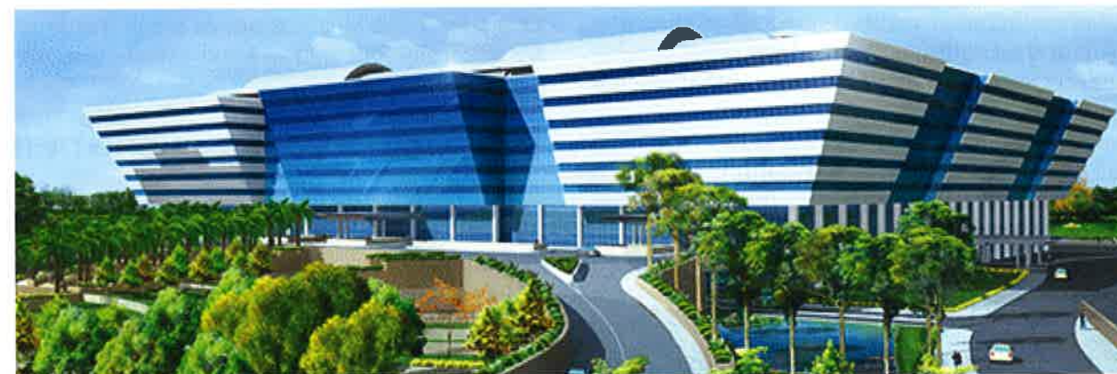
Bangkok Government Center, Post-Tensioned with Flat Duct Bonded Tendons (Courtesy PBL; P690)
