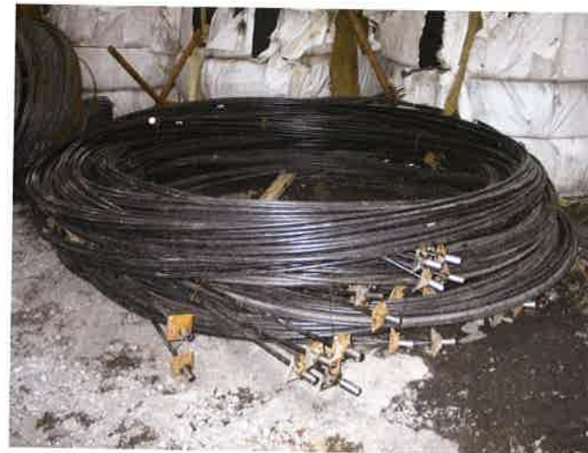
FIGURE 8.6-8 Delivery of Cut Strand to Job Site for Grouted Construction (Beijing; P727)
