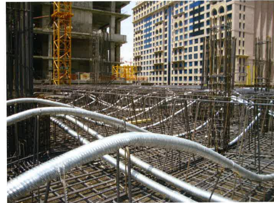
Transfer Plate under Construction (Jabal Omar Tower; KSA; P629)
