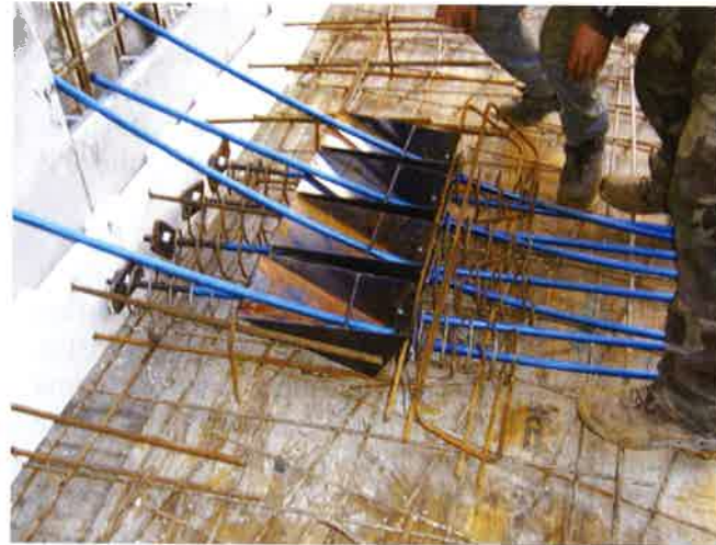
FIGURE 9.4-2 Stressing Pans at Top of Slab (Italy; P731)
