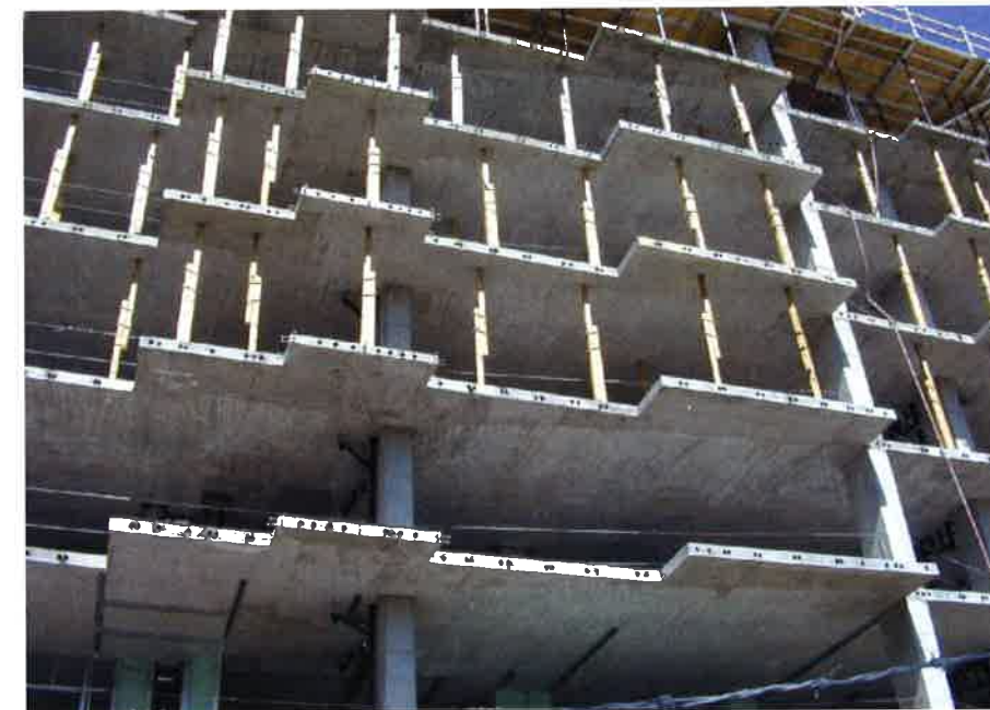
Post-Tensioned Concrete Frame under Construction (California, P634)
