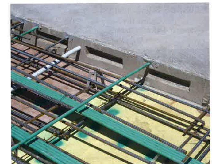
FIGURE 8.6-4 Construction Joint Unbonded Slab (US; P723)
