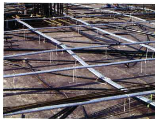
FIGURE 10.3.1-2 View of Tendon Layout Showing Wobble in Tendon (Tehran; P102)
