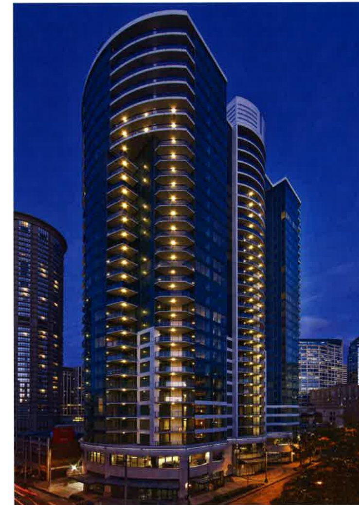
Post-Tensioned Multi-Story Building; Escala, Seattle (Engineered by Cary Kopczynski; photo by Michael Walmsley; P695)
