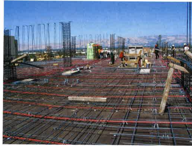
FIGURE 8.5.1-2 Reinforcement Layout of a Typical Floor (P114)
