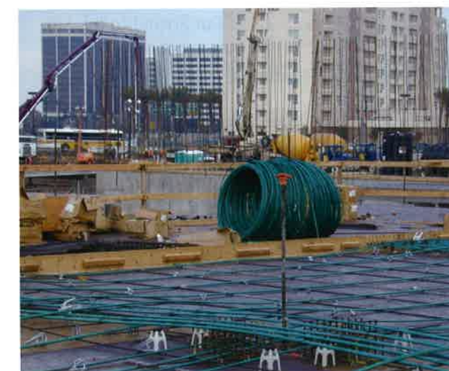
FIGURE 8.6-3 Unbonded Slab (UK; P722)
