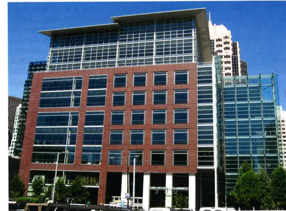
Post-Tensioned Building in San Francisco (Foundry Sq; courtesy Nishkian Menninger; P520)
