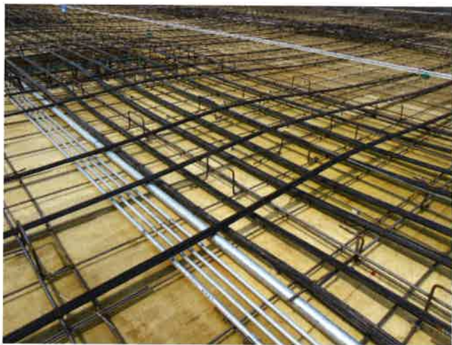
FIGURE 9.4-3 Unbonded Floor System (South Korea; Dailem P732)
