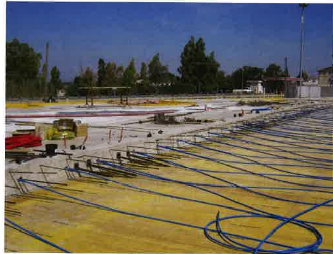
FIGURE 9.4-1 Construction Joint with Intermediate Stressing (Italy; P730)
