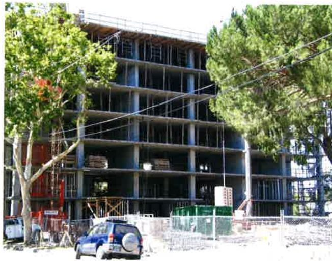
FIGURE 8.5.1-1 Building under Construction (P113)
