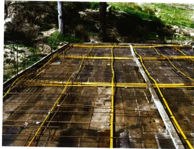
FIGURE 8.6-5 Unbonded Slab (La Paz, Bolivia; P724)
