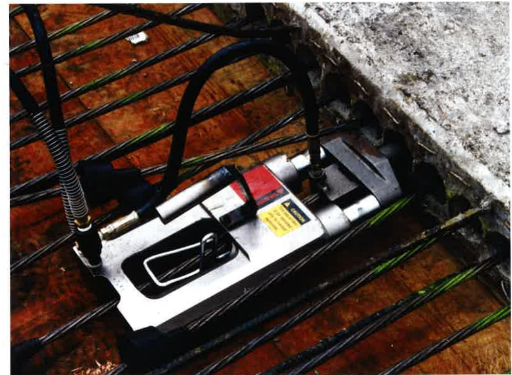
Tendon Stressing at Slab Edge (P607)
